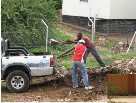
All building rubble was removed from the erf.
